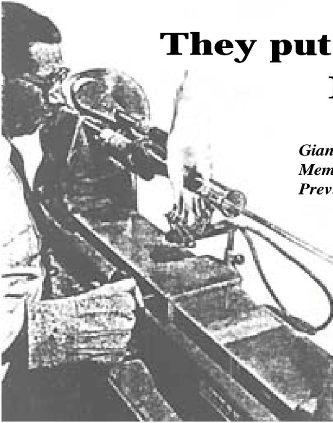
With yellow flame, James Ackerman, of Plant 2's Tube Manufacturing Dept., dries a coating on a memory tube for the 701.
